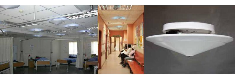
The Sani Disc Unit emits a UV-C intensity of approximately 10µW/cm<sup>2</sup> at a distance of 1,3m from the unit in a blanket of concentric circles (as per South African and International guidelines).
